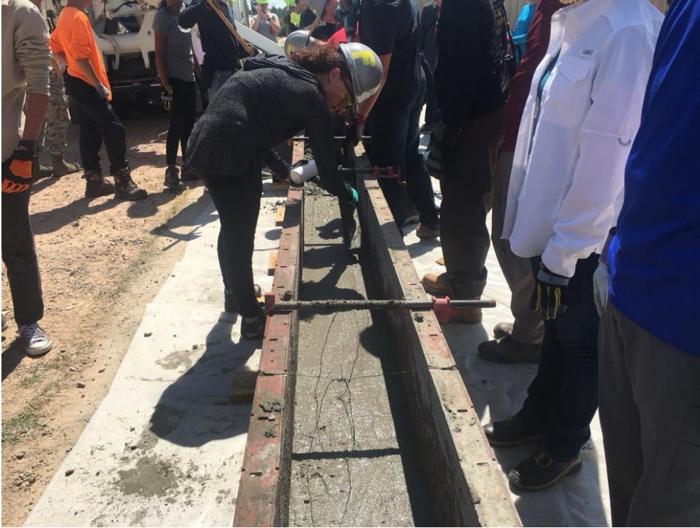
Me smoothing out our concrete beam.
